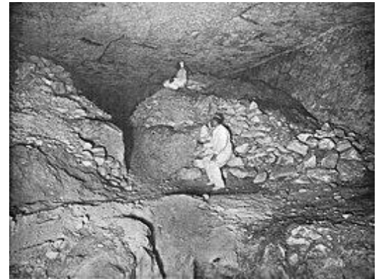
Subterranean Chamber (looking west) in 1909 with rubble from the Pit Shaft excavation still filling the chamber.
