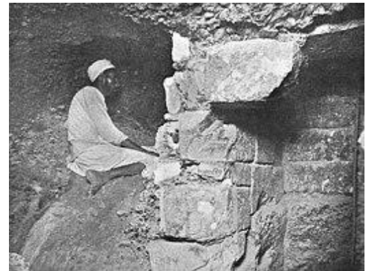
Grotto (left) accessed through the broken wall of the Well Shaft (right)
